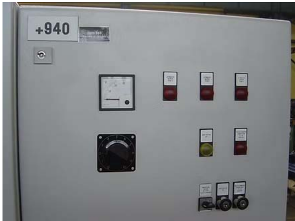
Steam testing unit electrical testing device (e.g. for a partial stroke test)
